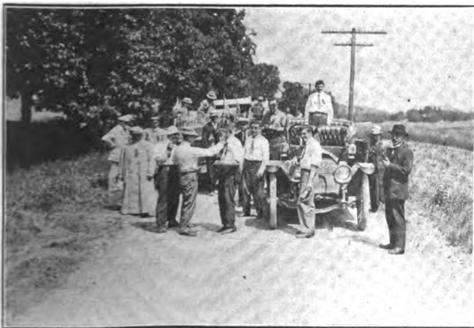
Inspecting McClintock's Cube Block Pavement near Charlotte
